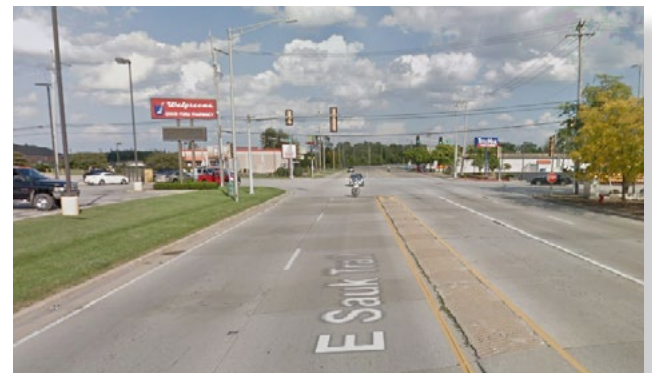
Existing intersection of Sauk Trail and Torrence Avenue.
