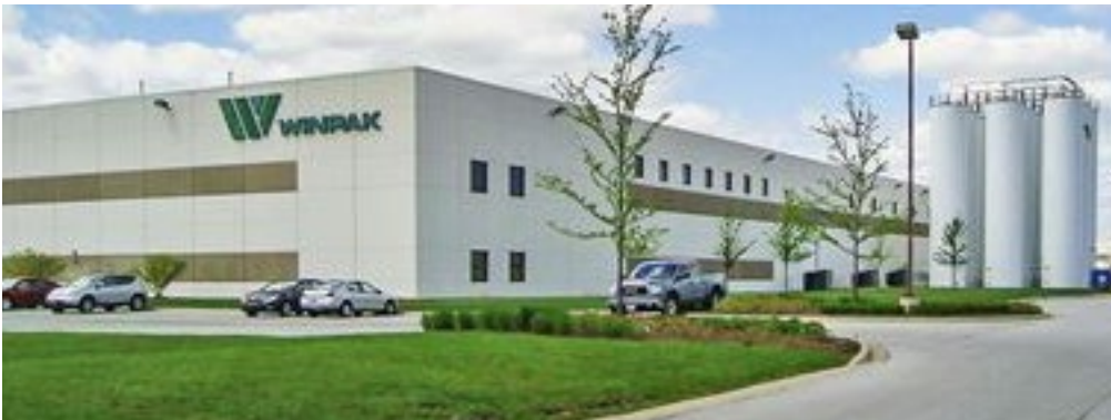
Winpak facility within the LogistiCenter.
