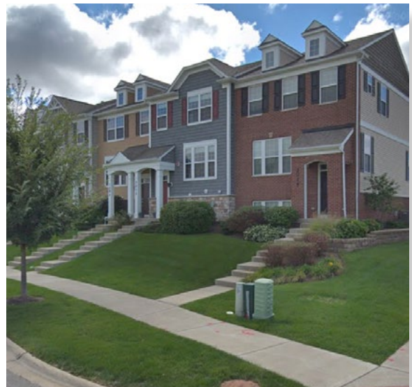
High-quality multi-family housing can attract a variety of residents to Sauk Village.
