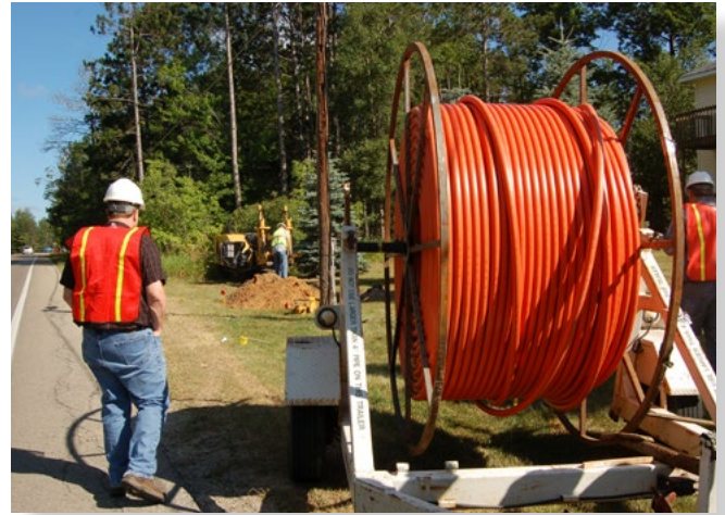
Installation of fiber optics expands development opportunity within Sauk Village.
